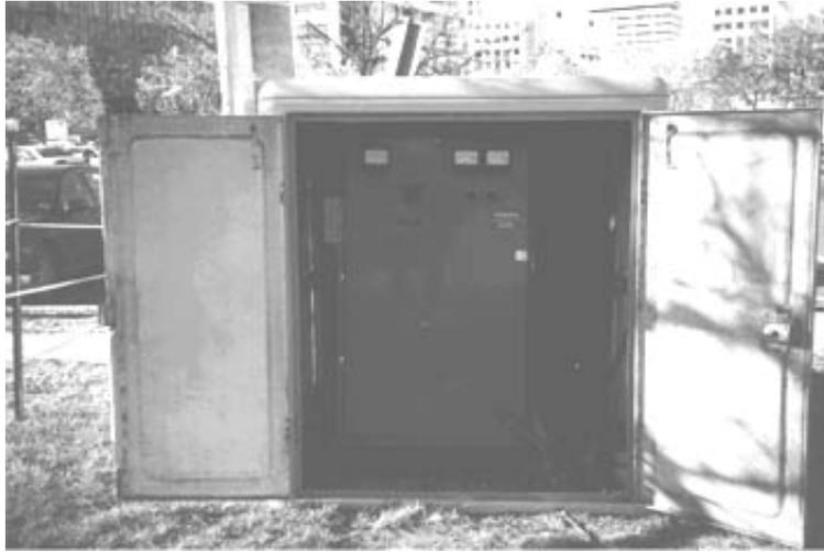
50A rectifier in weatherproof enclosure at Canberra
