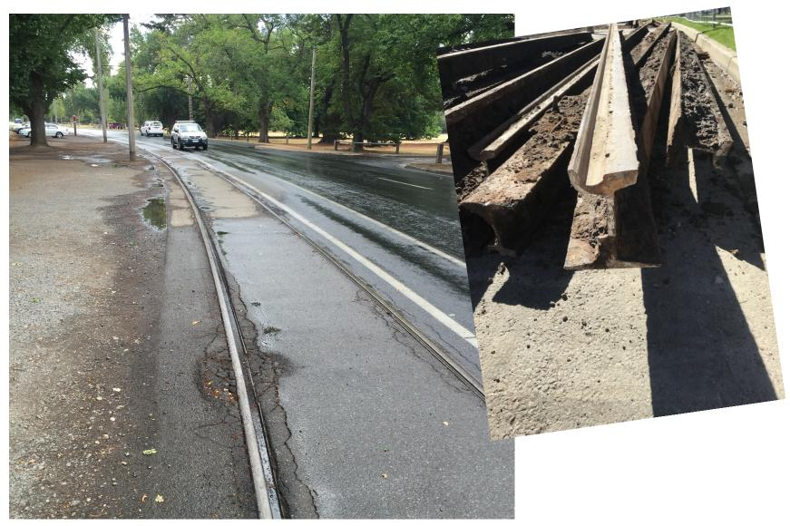
Track in Wendouree Parade had worn out—rails were between 80 and 115 years old. The road surface could not be maintained—poor sleeper (if any) condition.
