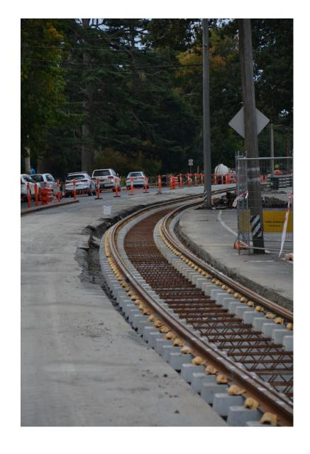
Work commenced on 2 April 2022 with commissioning on 25 August 2022, after a very long wet weather period when doing the trackwork for the new Museum, Included was the installation of new poles and overhead work. The ride is now very smooth—no bangs, crashes and much less swaying.
