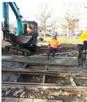
Photo: Tony Weston Concreting of replacement point work.
