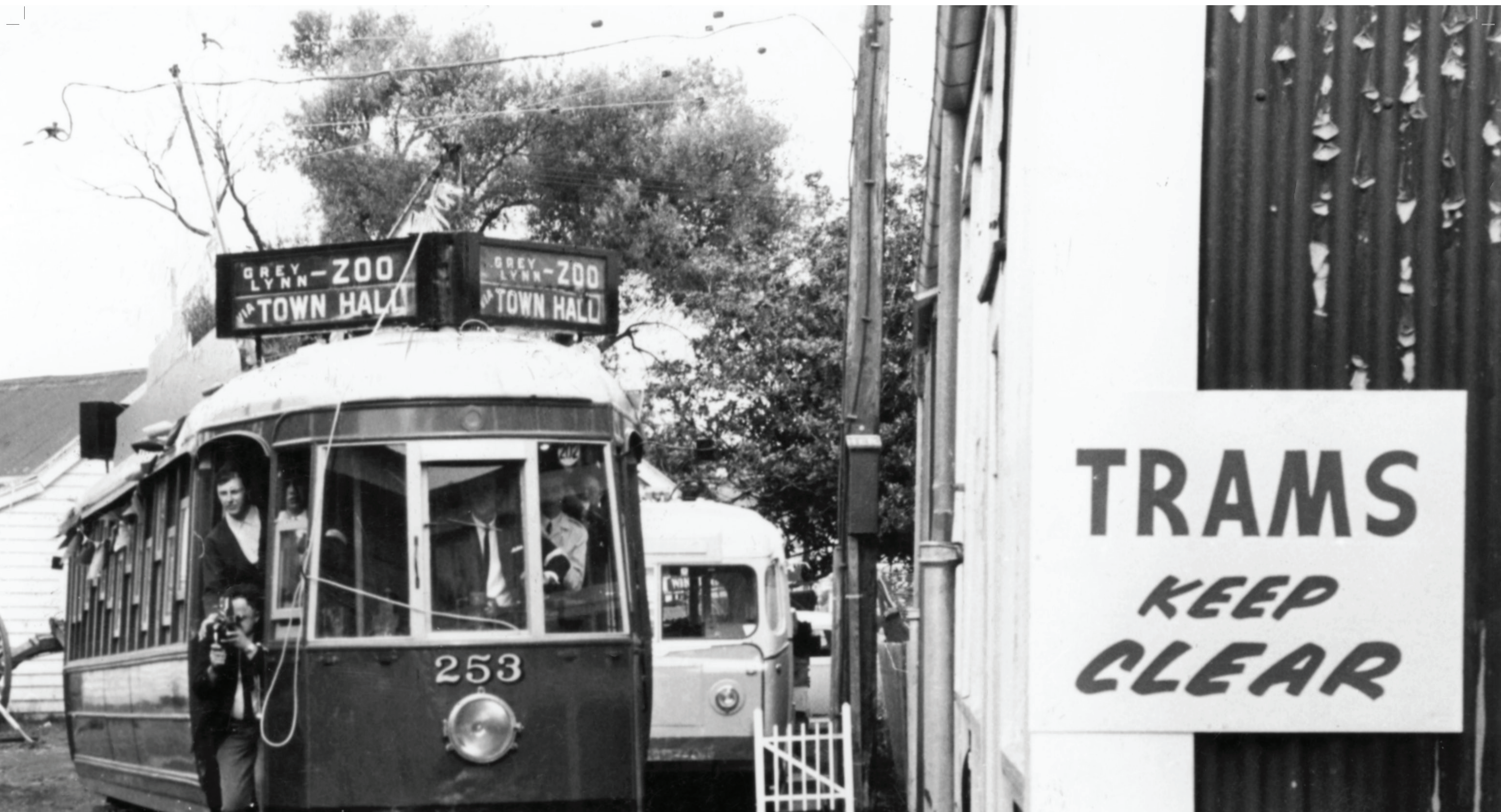
Image taken opening day of the tramway, showing the feeder cable above the tram connected to the running wire. The box fixed to the wooden traction pole on the far right has the knife switch installed that controls the feed from the trolley bus system.
