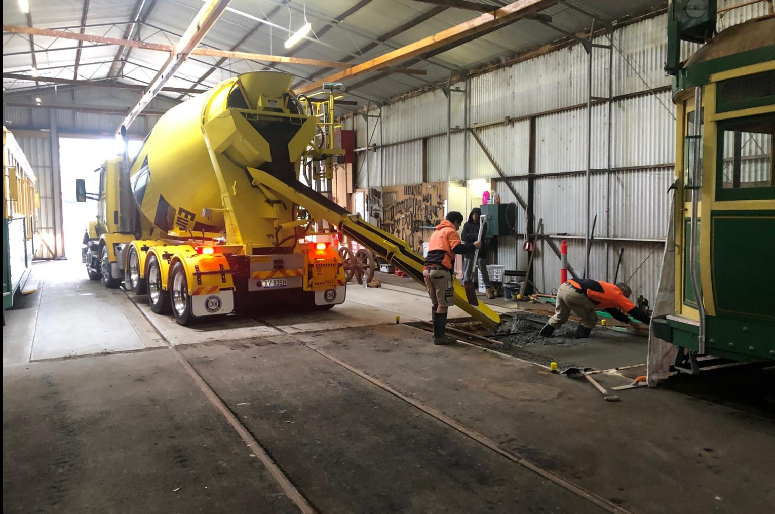
Pouring concrete within the carbarn
