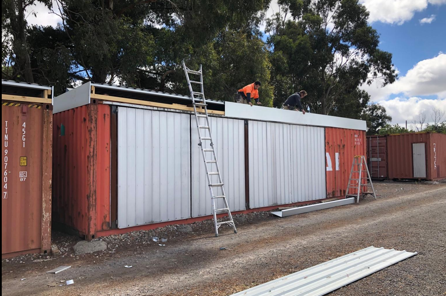
Provision of roofing over 40-foot shipping containers
