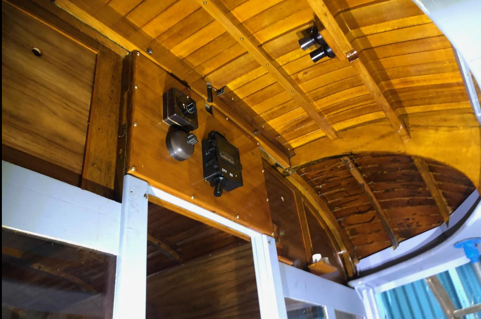
Overhauled line breaker and lighting switches installed
