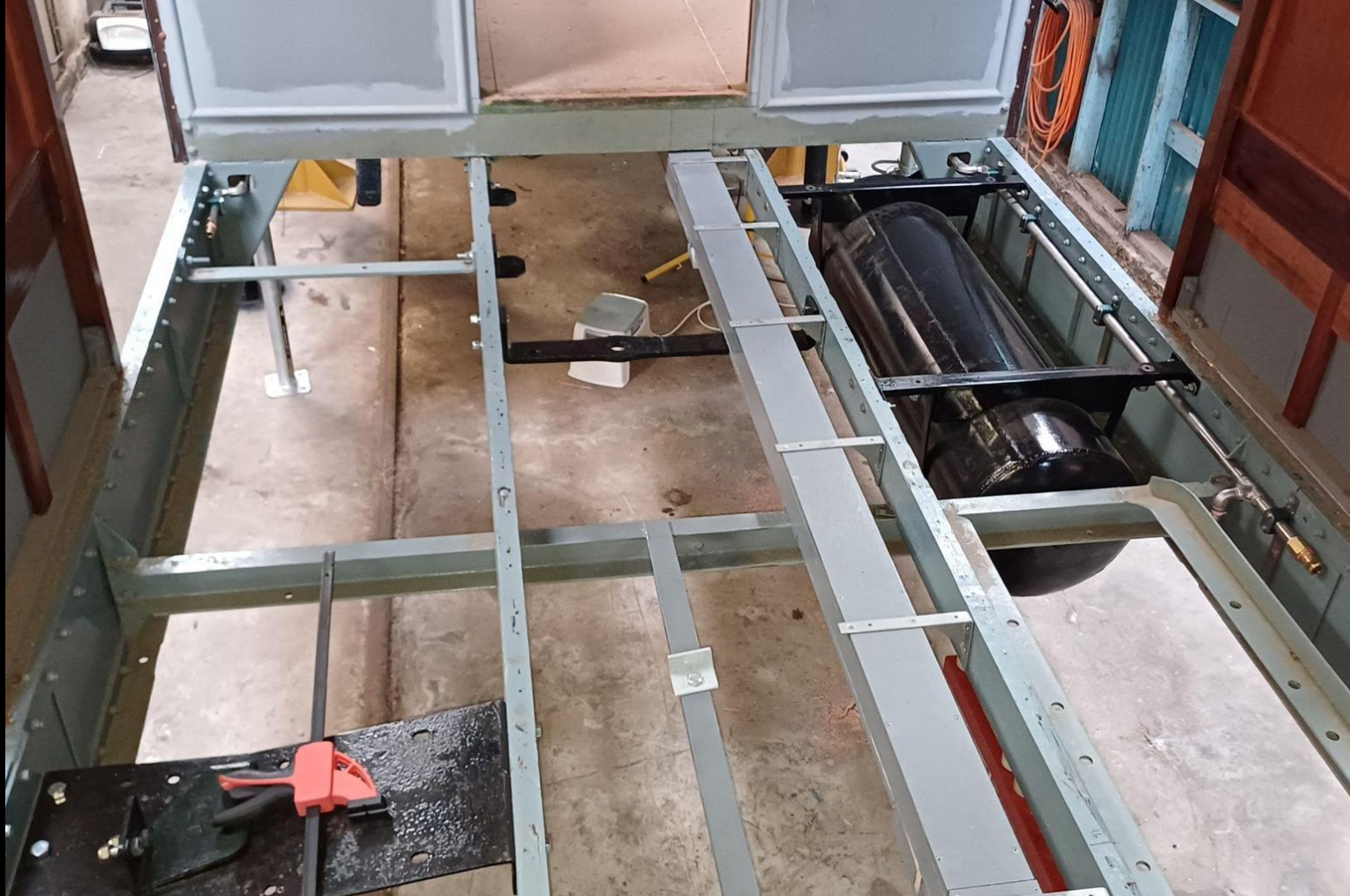
Installation of underfloor reservoir tank and pneumatic piping
