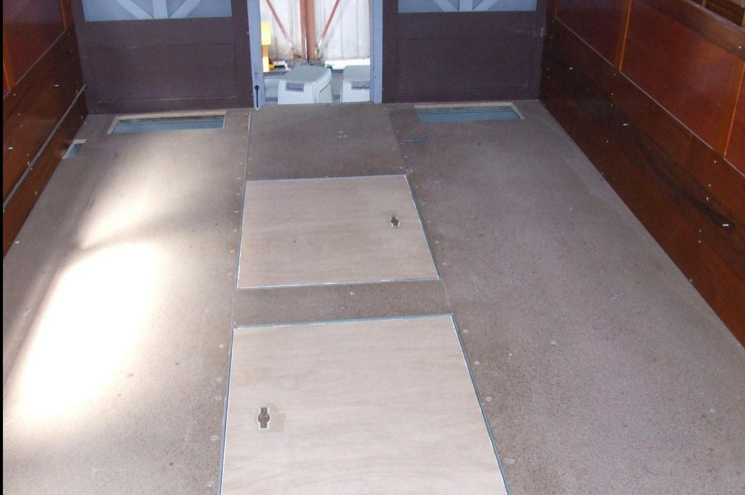
Completed saloon floor
