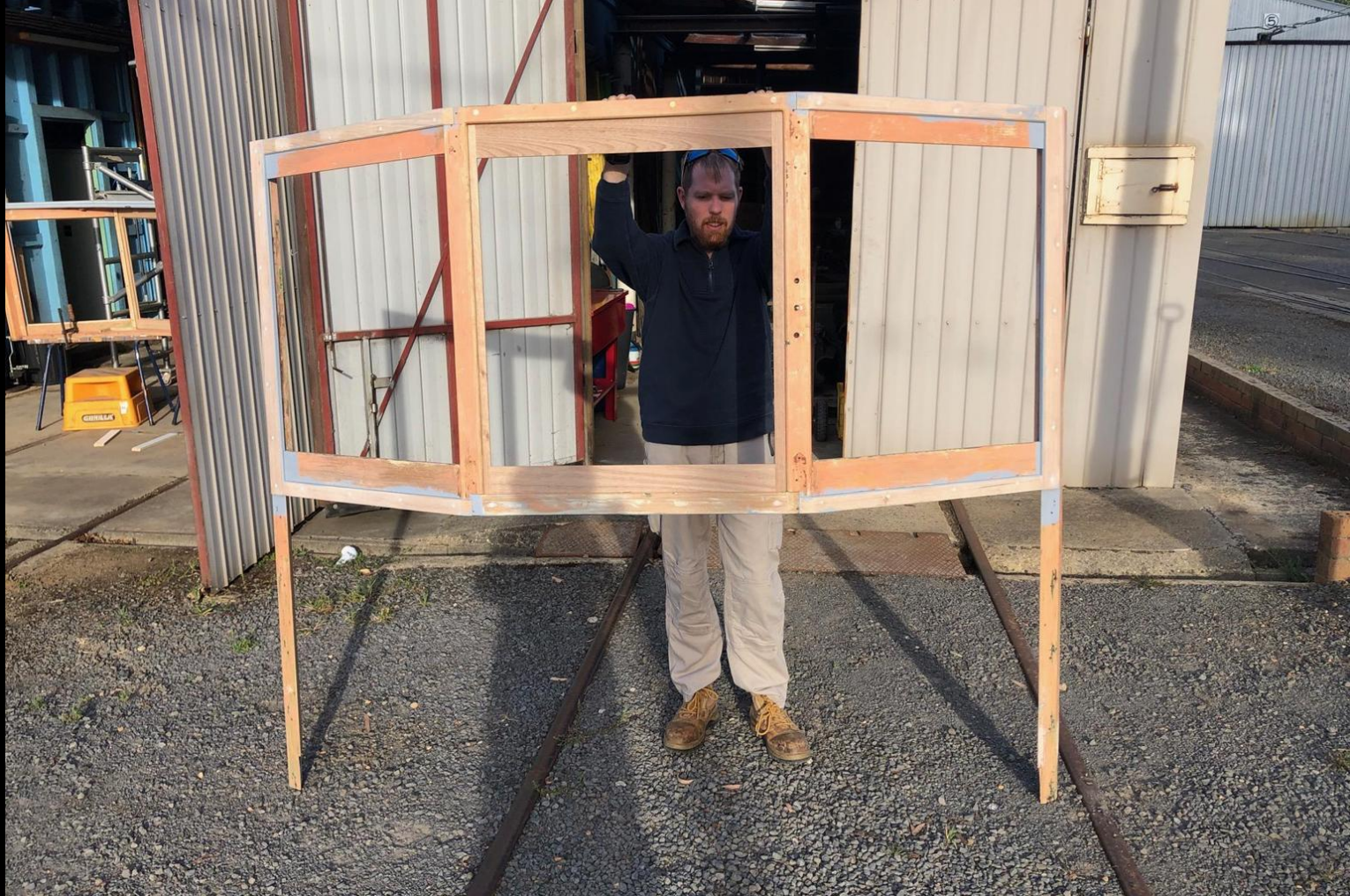
Daniel holds up one of the completed windscreen frames prior to installation
