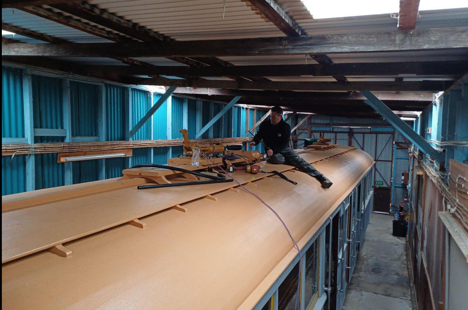
No harness needed! Clinton installing cabling on the roof of 792
