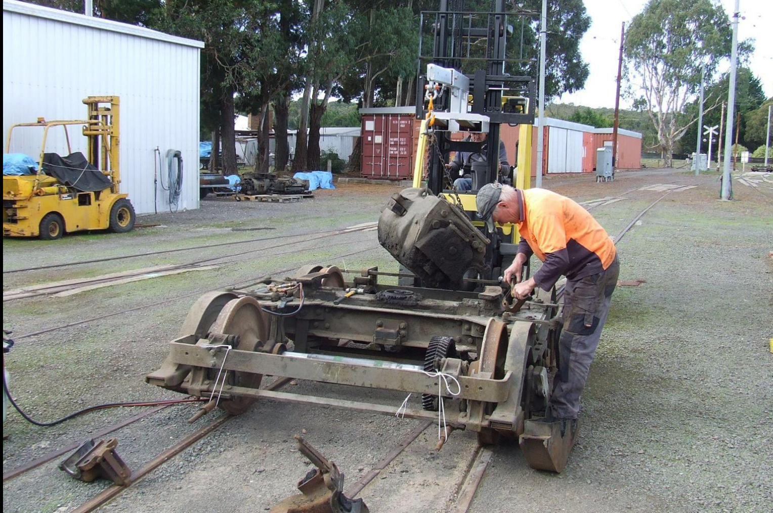
Dismantling surplus trucks to provide spare parts for other COTMA groups
