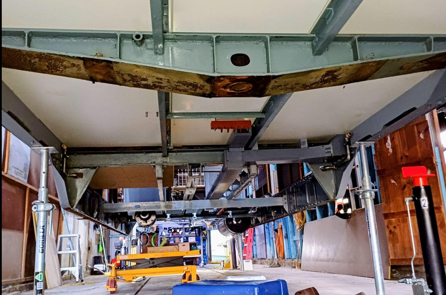
Body of 792 supported by new hydraulic stands
