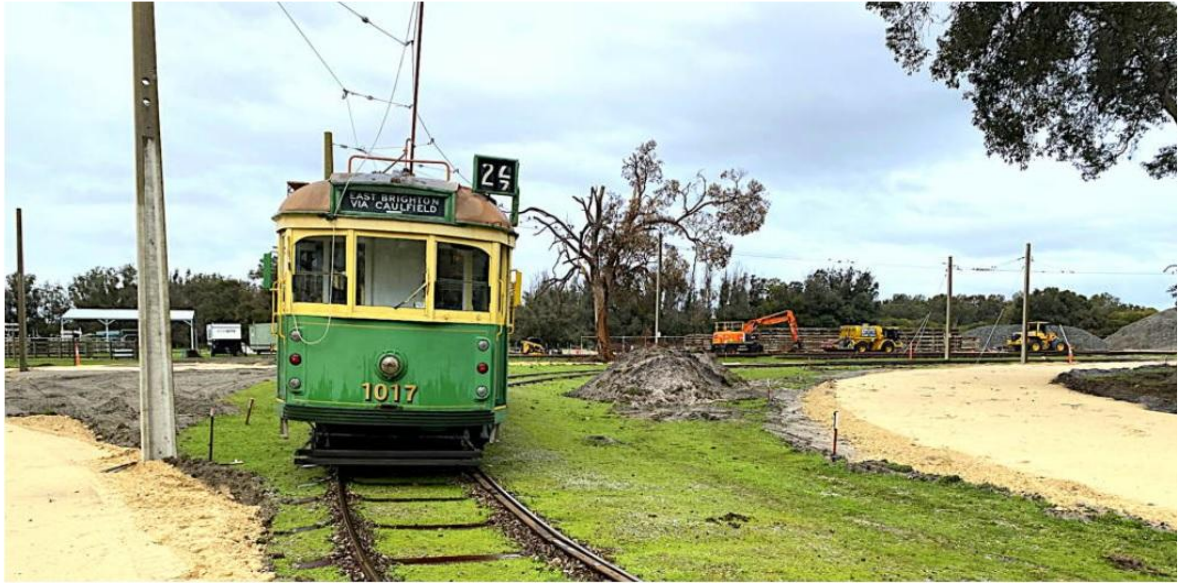
On the last weekend of service before shutdown, W7 1017 is surrounded by track works as it passes along what is left of the triangle.
