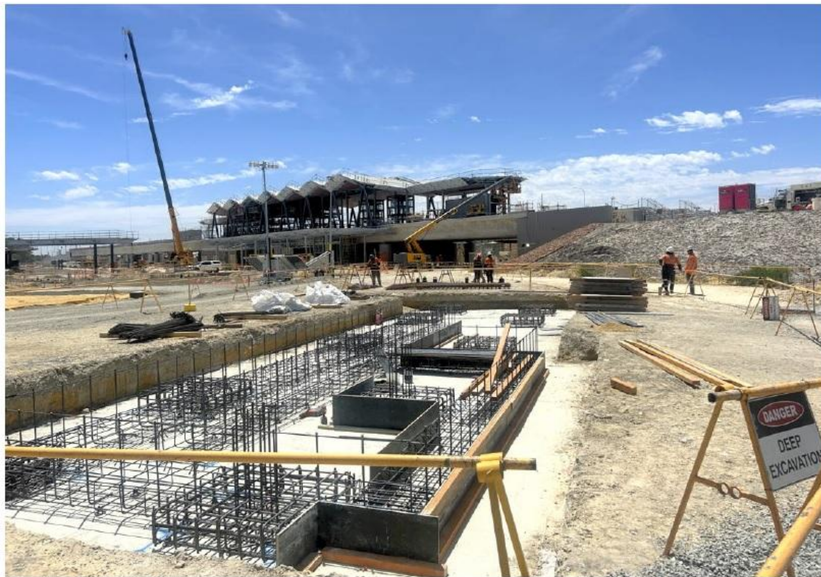
The new tram terminus under construction in the foreground, and Whiteman Park Train Station nearing completion in the background, on 20 February 2024.
