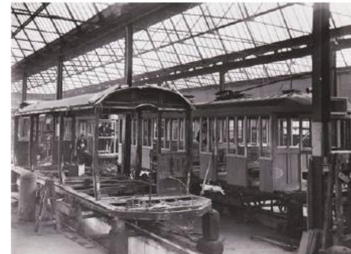
Conversion of L class tram to L/P at Randwick Tramway Workshops
